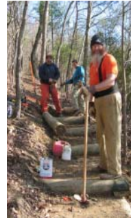
Community members construct a portion of the trail
